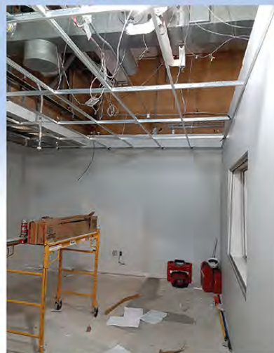
Drywall is installed.
